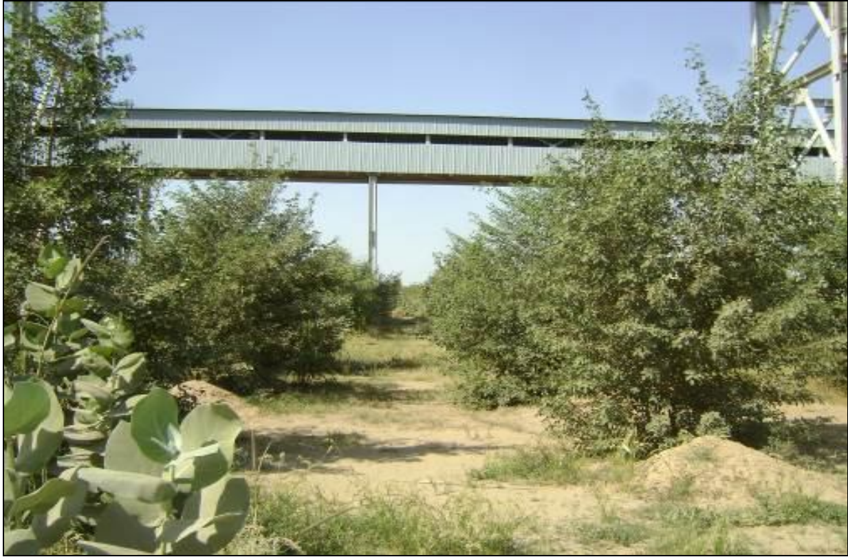
Location: Greenbelt Nr. Conveyor Belts
