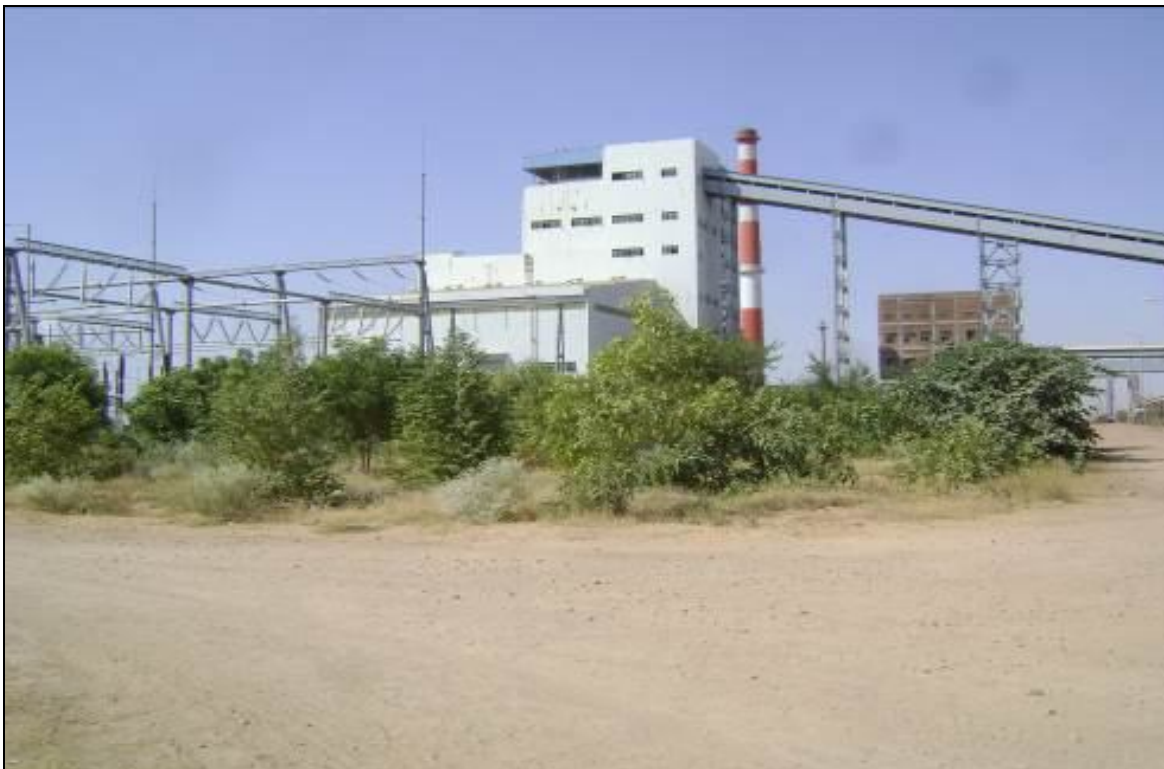
Location: Greenbelt Nr. Switchyard with clear chimney at full load
